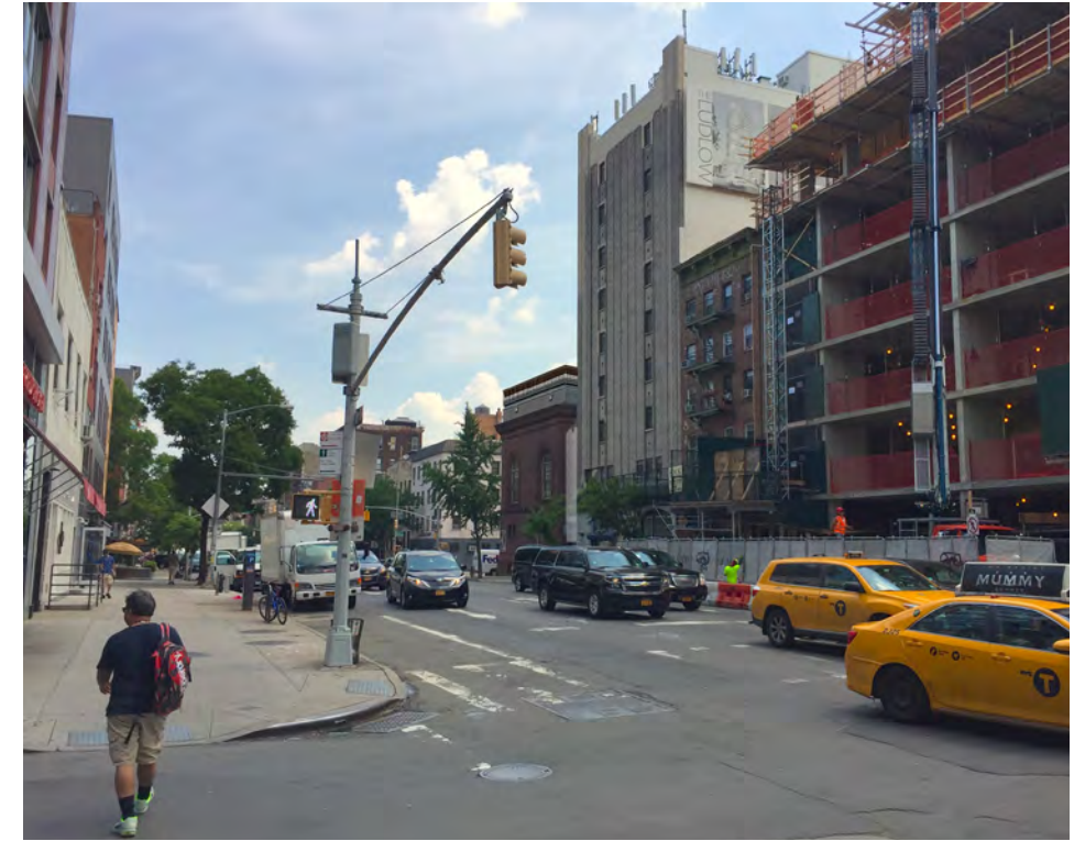
VIEW FROM 2nd AVE LOOKING NORTH
